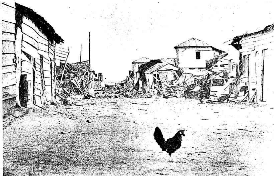
Bomb damage at Massana. 70,000 people were left homeless.
